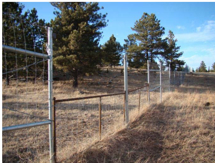
Figure 11. Photo of double wide elk jump gate in lowered position (Photo Credit: Wind Cave National Park).
